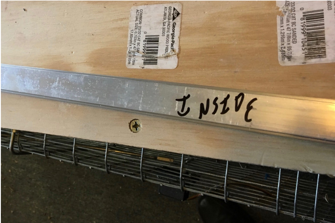
Figure 5: Mark exposed side of Strip to prevent it being flipped causing a misalignment
